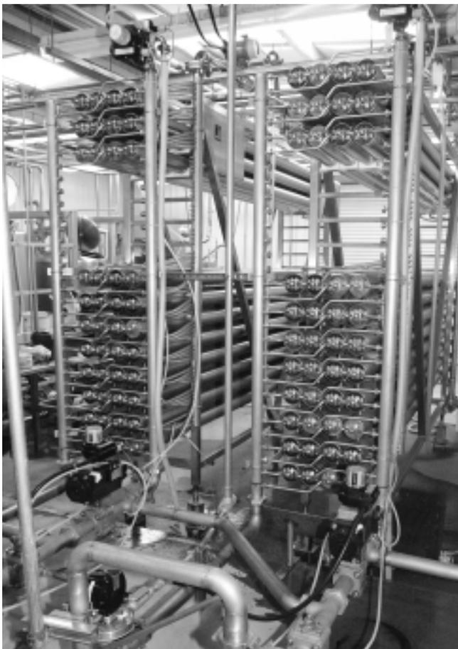
*This membrane filtration plant incorporates 80 filtration modules and is designed so that it can be easily expanded 50 percent to 120 modules to meet increased demand in the future.*
