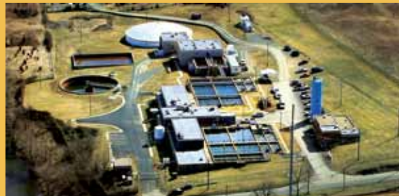
The facility uses two different treatment processes to produce potable water.
