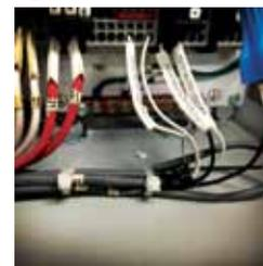
The next step is to verify that the electronic control panel has been wired correctly by a certified electrician. All control panels should include a wiring diagram for the electrician to follow. A few of the expected wiring requirements are main power supply connection, solenoid connection(s), sensor connection(s), remote set point connection(s), alarm(s) and remote control input connection(s).
