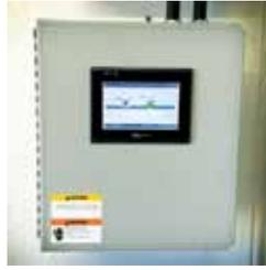
Ensure the sensor value(s) match the signal(s) displayed on the electronic control panel. If there is a considerable discrepancy between the values, this is often because of a range mismatch. If there is a minor discrepancy, this is usually because of the zero and span calibration values compared with the incoming sensor signals. To rectify these issues, repeat step 6 until values are accurate.
