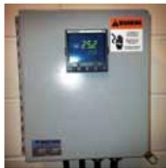
When the solenoids and the sensors are verified, the next step is to start using the electronic control panel to its full potential. Before releasing the panel to control the valve automatically, follow the manufacturer's user manual on tuning process for setting up initial tuning control values. Once set, introduce a small
