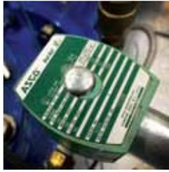
With power now available, the valve solenoids can be energized and tested. Before testing can begin, the solenoid orientation needs to be set up within the electronic control panel.
