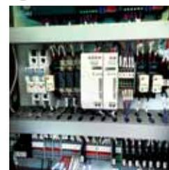
Flip the breaker on the panel to start the electronic control panel. The screen and controller should turn on. If additional parts are included in the panel, check that the power supply, uninterruptible power supply/battery system and filters are functioning as needed. This usually is indicated by a "System OK" or "DC OK" indicator.
