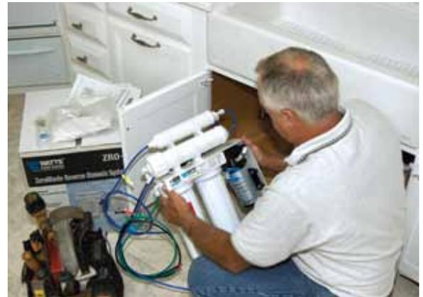
to faucets and showers. An RO system also may be installed as an additional step for treating water.
