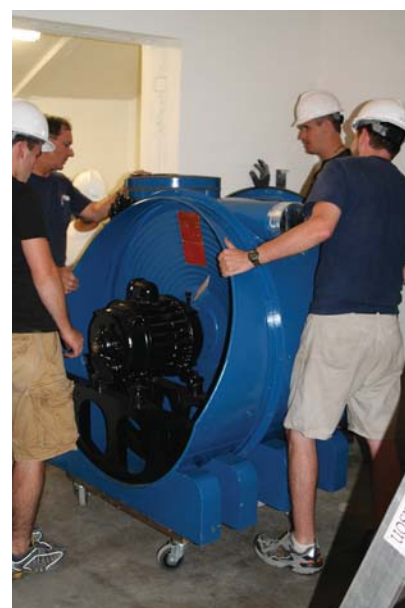
FBI techs guide the blower into the new blower room.
