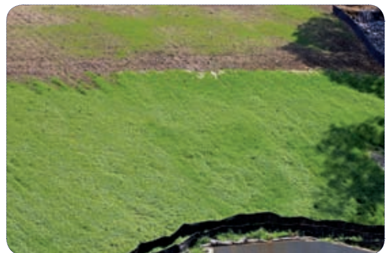
Roadside slopes on which the cotton fiber-reinforced matrix was applied held up well during severe rain events.
