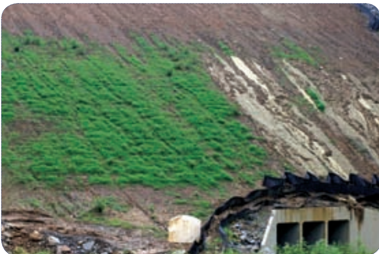
Roadside slopes on which the cotton fiber-reinforced matrix was applied held up well during severe rain events.
