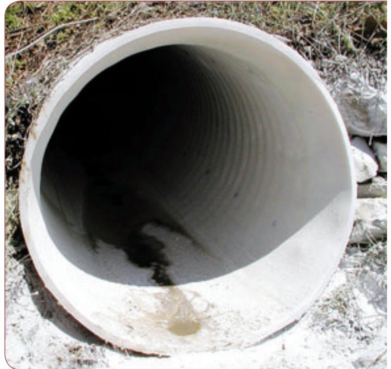
County officials consider factors including cost and resident impact when assigning projects to CIPP or open-cut contracts.
