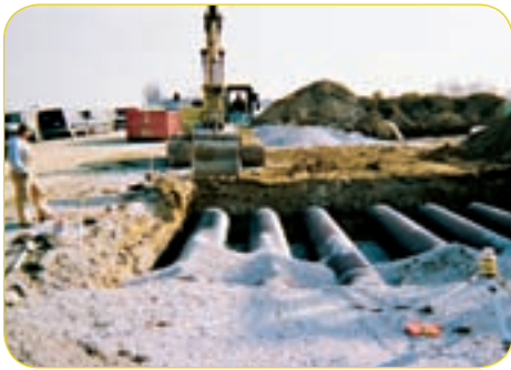
Subsurface storage systems can save valuable real estate.
