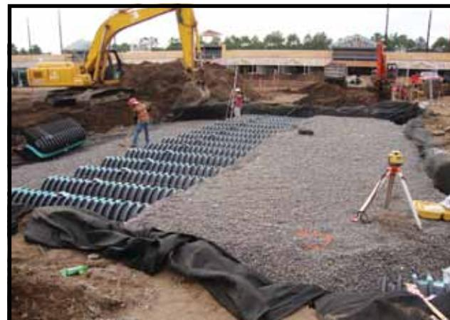
According to the engineer, this system was the solution due to ease of installation. Cultec employed its own in-line side portal manifold, eliminating the need for a costly external pipe header. Such a system was easier to install than a conventional manifold system and also was more cost effective. Additionally, the system used less stone than other comparable systems on the market and required no heavy installation equipment.
