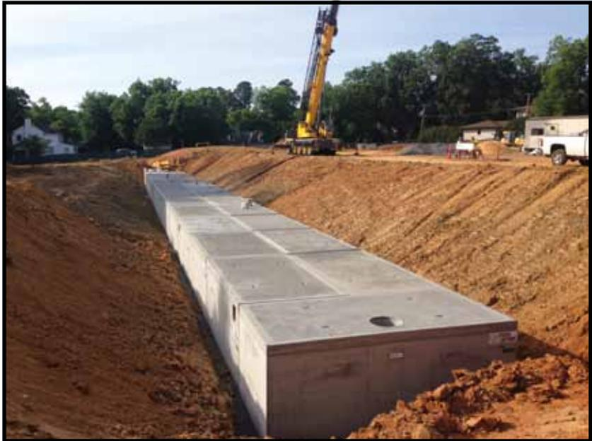
first day. On day two, the modular nature of the system provided the contractor with an opportunity to easily install all of the internal sand filter components (under-drain piping, stone and sand media) while the system was still open. On day three, the tops of the modules were installed and backfilling operations began. The Cottages project is scheduled to have townhomes available for occupancy in January 2015.
