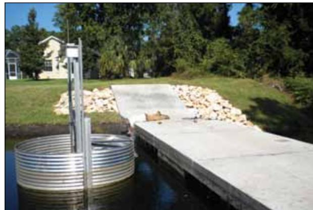
**Top: The pulse inputs connected to the tipping bucket collect rainfall data, while the analog outputs control the canal gate. Bottom: Control structures with electrically actuated gates regulate flow in the canals.**
