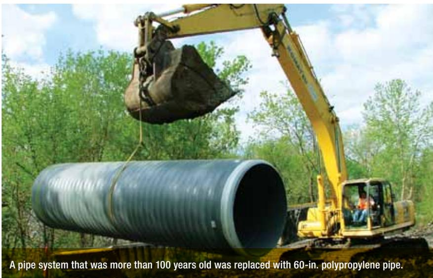
A pipe system that was more than 100 years old was replaced with 60-in. polypropylene pipe.
