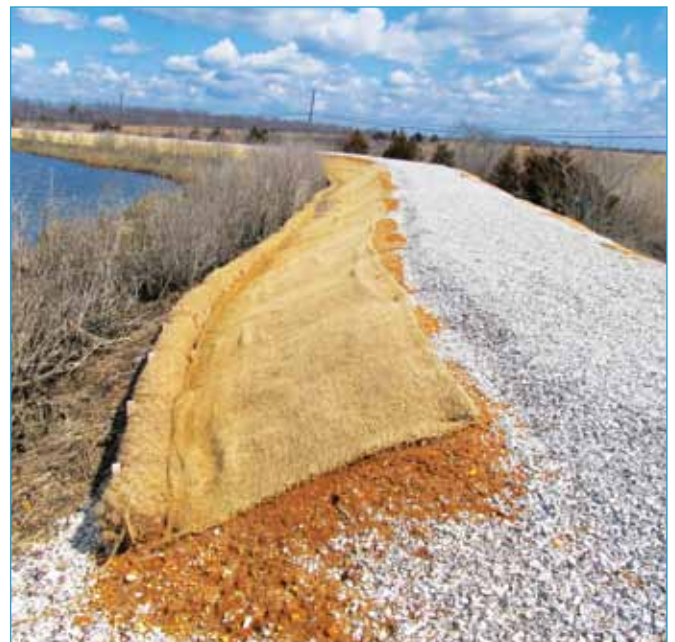
The coir log installation
