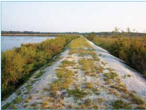
The dikes now are fully repaired with the coir products installed.
