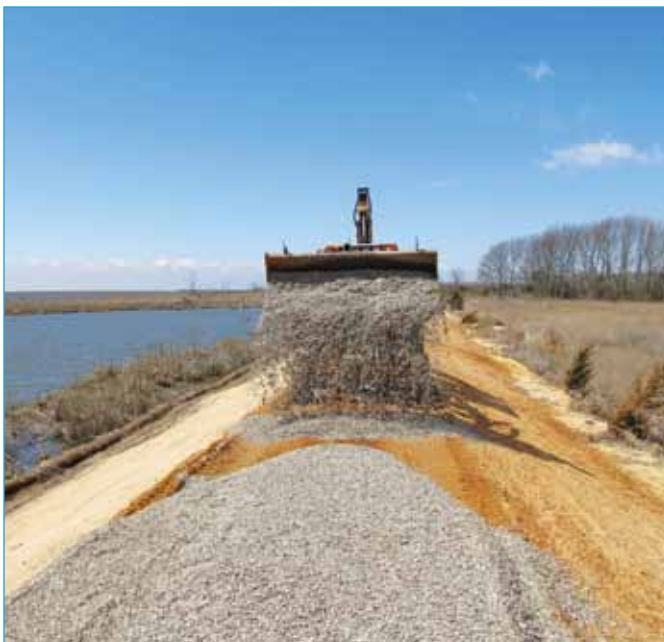
A road made of crushed seashells is laid.
