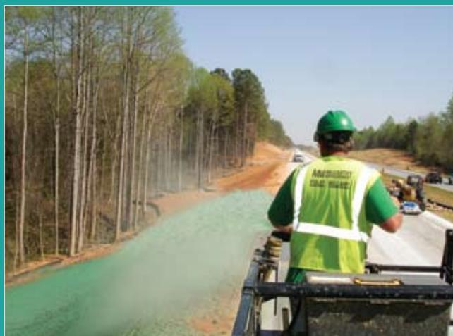
Left: SCDOT's \$60-million rehabilitation of a stretch of I-385 called for an arduous erosion control task to keep soil from eroding in areas dissected by two dozen streams. Right: Vegetation is applied to 300 acres of steep slopes, much of it during the heavy rains of winter and spring.
