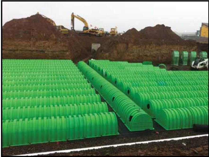
sediments onto a special floor that is easily accessed and cleaned, the main header row distributes water to long storage rows, where it is held and leached through a special glycol treatment zone before being released to the existing retention area.
