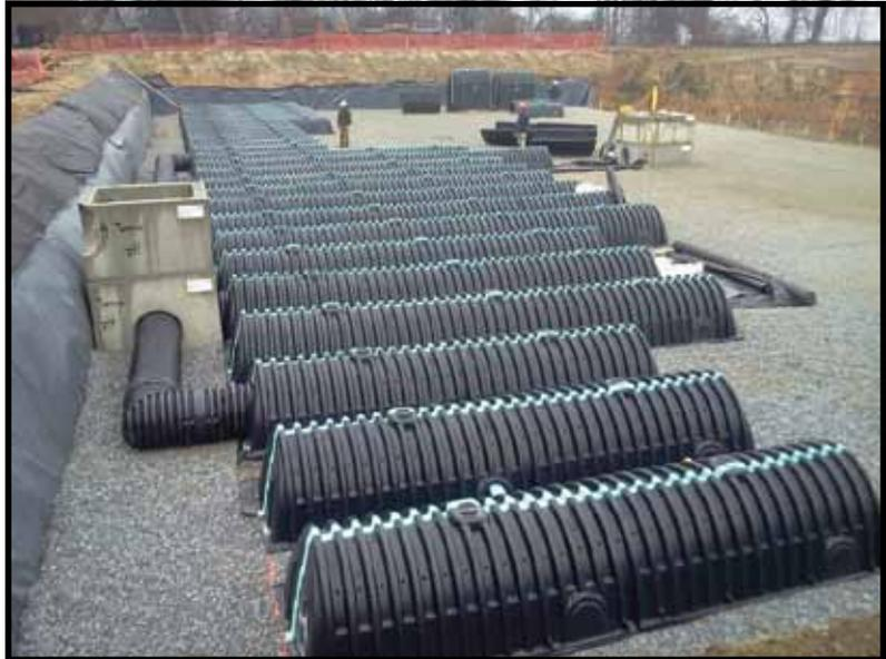
chamber can help save land space and offer design flexibility. In all, the subsurface system provided 94,319 cu ft of storage.
