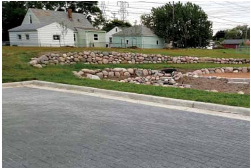
The parking lot's permeable pavement system includes a water harvesting system that overflows into a storage reservoir for irrigation of the orchard and hoop houses.
