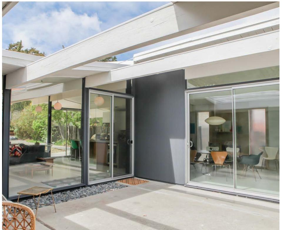
Aluminum is not recommended in beach homes for while the material is water resistant, it can suffer corrosion from salt water and salt air. The corrosion affects hardware operation and frame performance.
